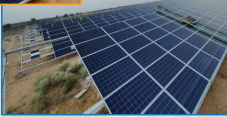
Robots used for cleaning solar modules
