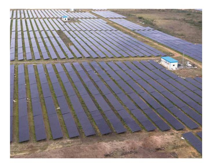
We were able to develop a Seasonal Tilt design which does not cause any damage to fragile thin film modules during tilting while keeping the cost of the structure low and increasing power output.
